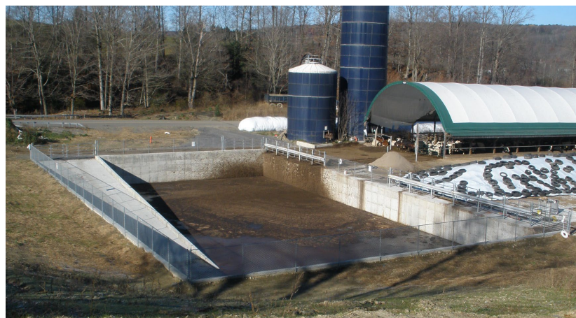
Completed waste storage facility
