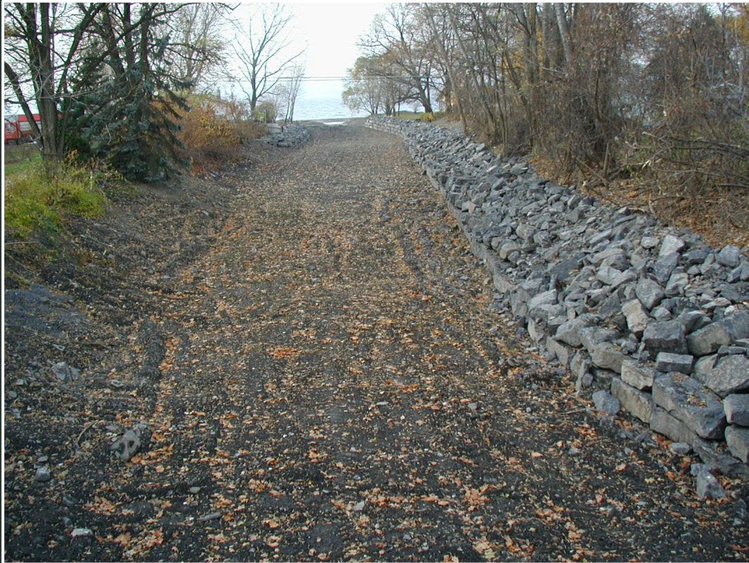
Mill Creek – Streambank Stabilization 2007
