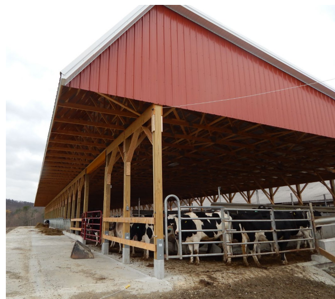
Completed Covered Barnyard
