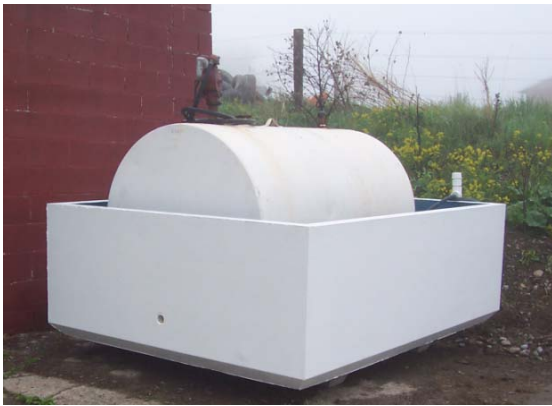
Example of fuel containment vessel that will be purchased with grant funds.
