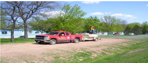
Below: Phil Griswold hydroseeding along Routes 5 & 20
